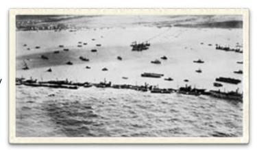
The Corncobs were to be sunk in two and a half fathoms or less at mid tide. That allowed the hulls of the ships to provide good protection for the beaches and small craft anchorage while leaving the superstructures above water and available for other uses.
